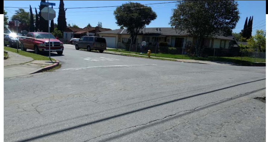
Florence Ave: PCI 51, 2004 Chip Seal
